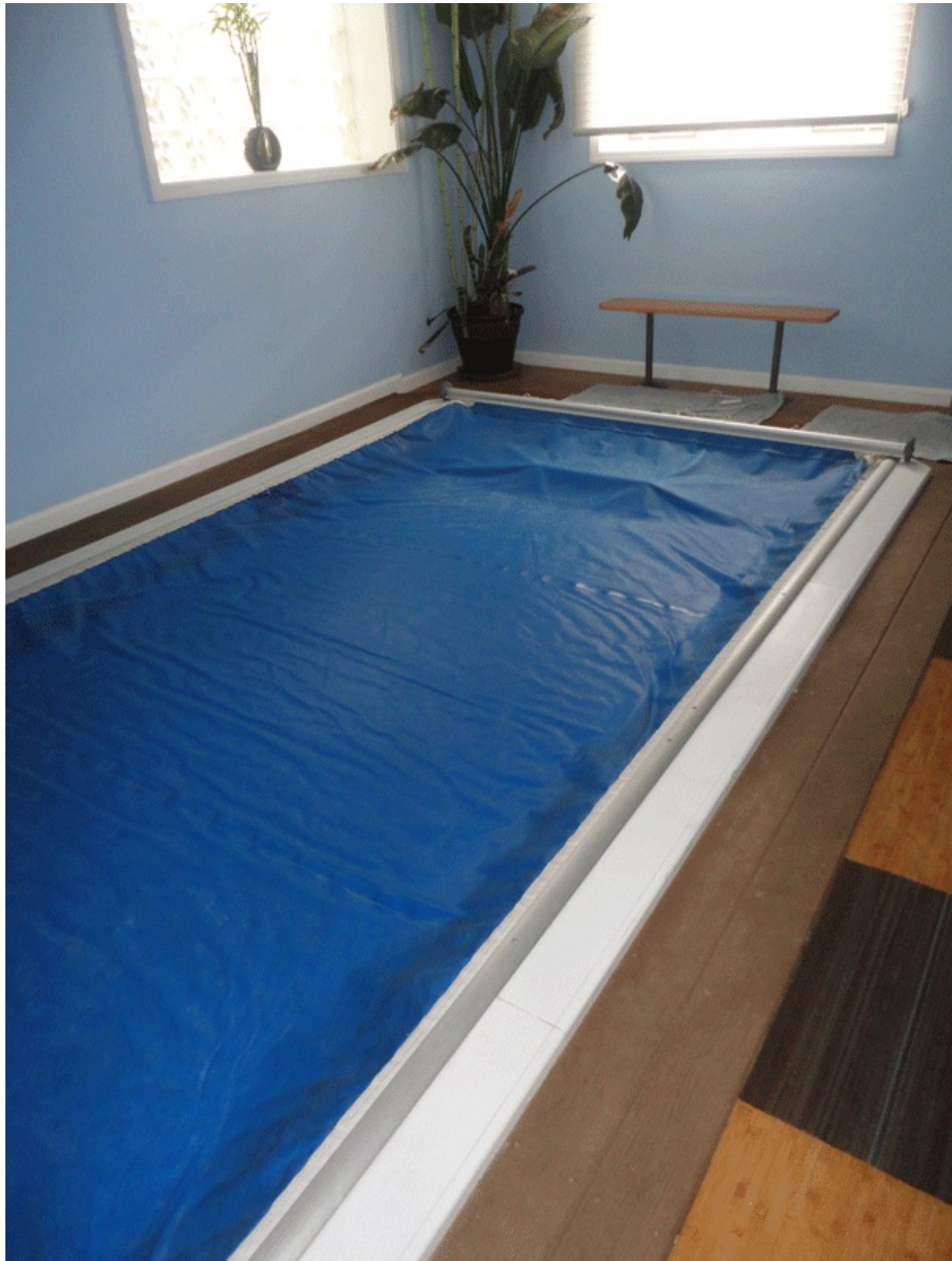
The basement swimming pool – since repaired – was for a time filled with raw sewage.
